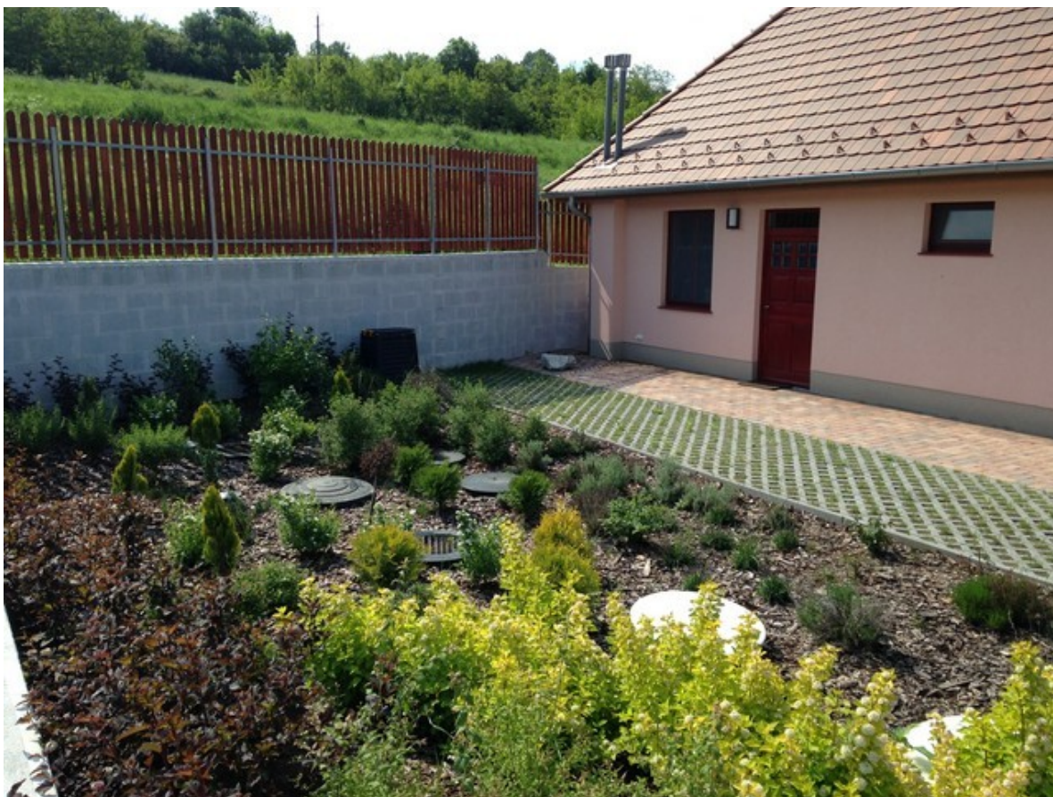
Picture 5: Waster water treatment and rainwater storage.
