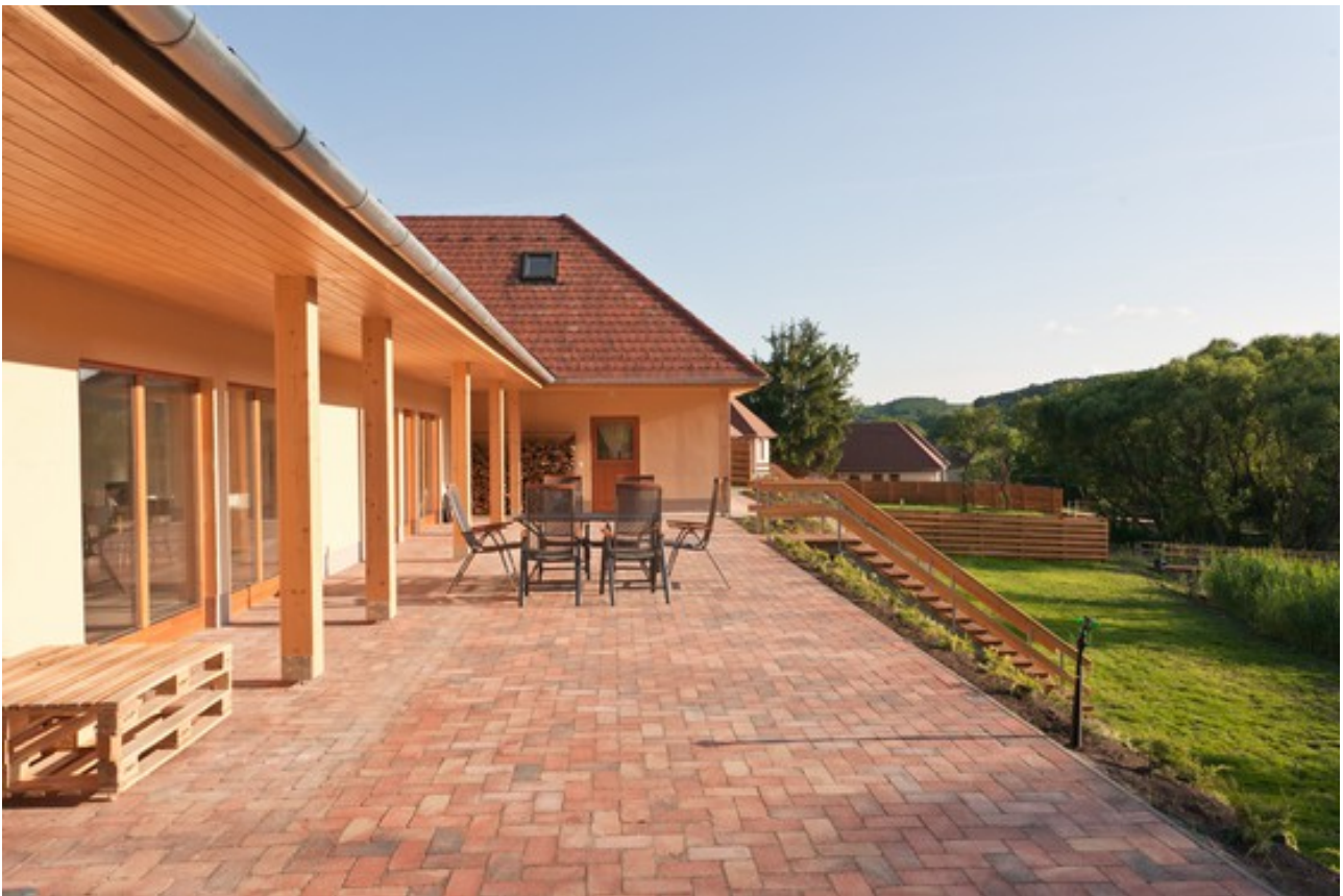
Picture 1: Terrace of the Upper House
