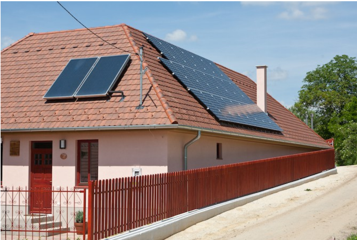
Picture 3: 6.56 kWp photovoltaic solar system (right) and solar collectors (left) at Irota EcoLodge Middle House.
